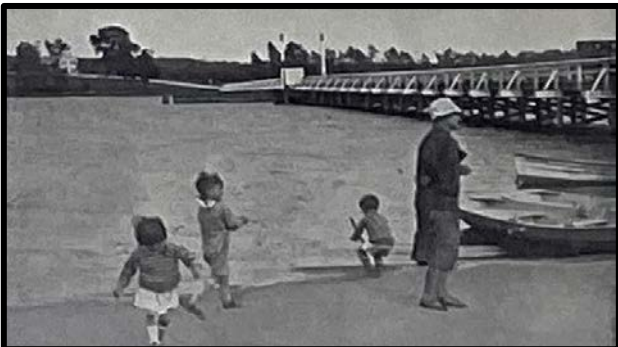
(above) The Allen Osborn Bridge constructed circa 1850. This photo is copied from the sales brochure of development brochure of Riviera Beach in Brick Township circa 1930.
