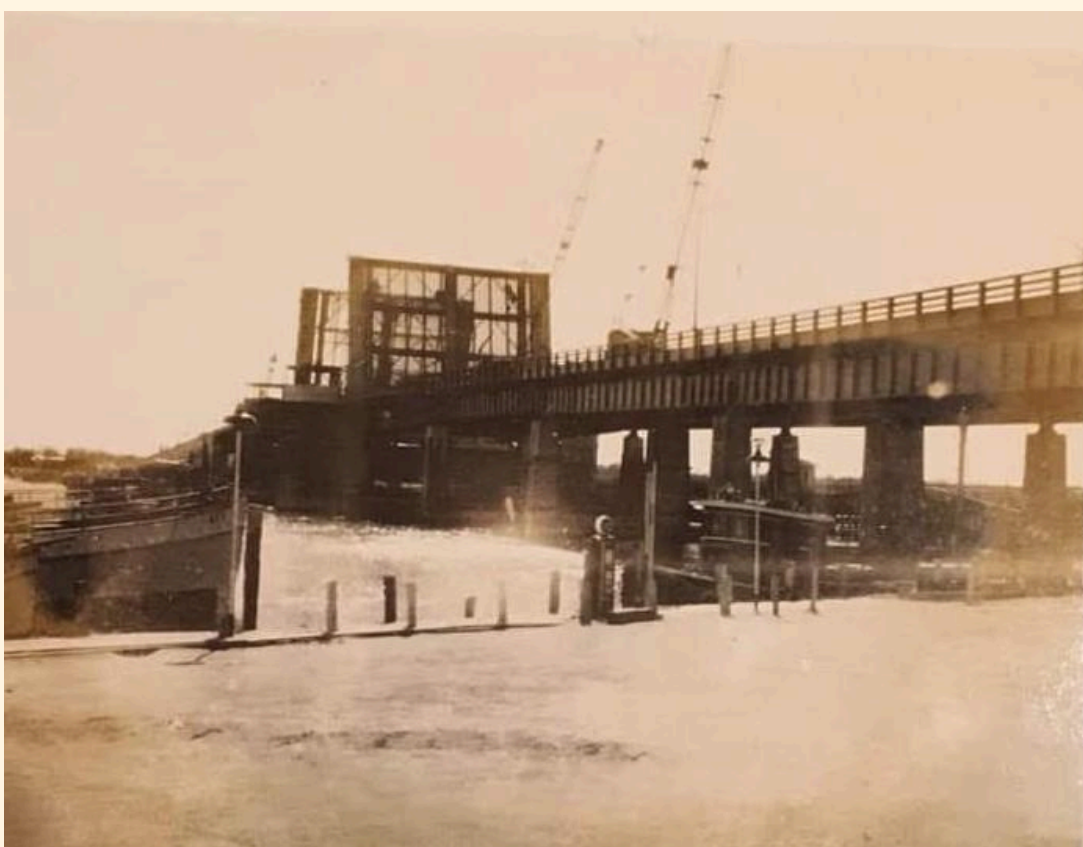
(above) The current Highway 35 Bridge nearing completion in 1952. The view is from Bogan's Basin in Brielle looking toward Point Pleasant.
