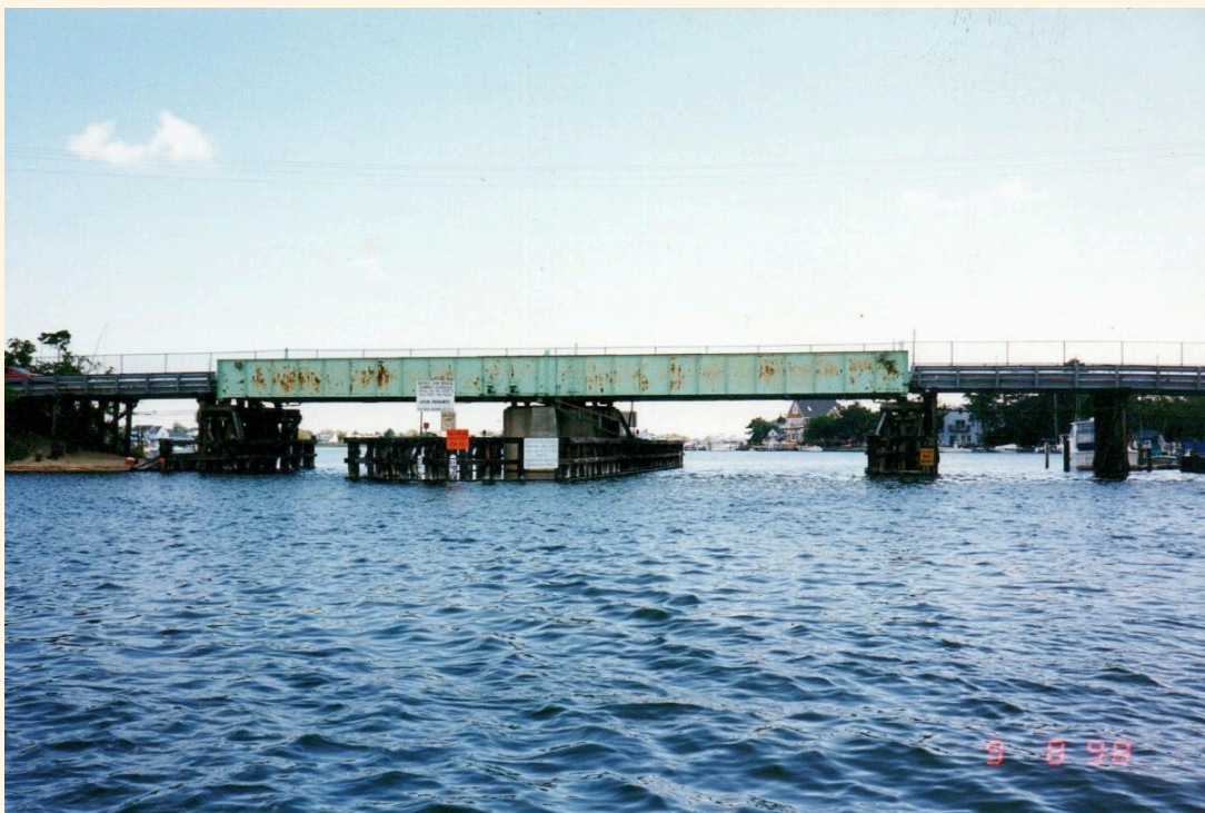
(above) A 1998 view of the Beaver Dam Bridge with a steel, swing center span. This bridge was replaced in 2000 with a lift bridge still in use today.
