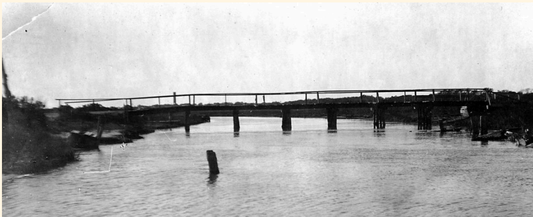
(above) The original "wagon bridge" provided access over Cooks Creek to the inlet area via Cooks Road, a diagonal route through the Cook Estate acquired by the County for pedestrian and vehicular access to the inlet..
