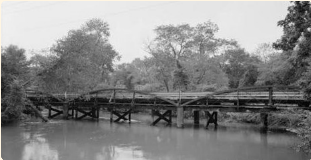
A view of the former "Squan Bridge" which was one of the first bridges to cross of the Manasquan River. The bridge was built c1887 over a narrow section of the Manasquan River at Lakewood Allenwood Road.
