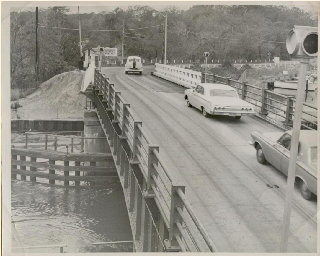
(above) A view of the old Lovelandtown bridge looking west. An iconic structure with its center swing, steel draw. In 1960 Police Chief William Beecroft warned that the then 33 year old structure was unsafe for vehicular traffic.
